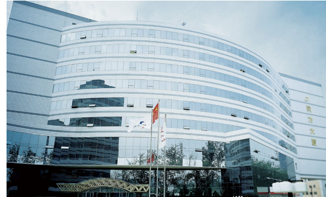
MIYUN MANUFACTURING BASE
