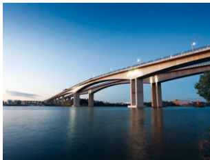
Gateway Bridge, Australia
