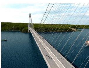
Third Bosphorus bridge, Turkey
