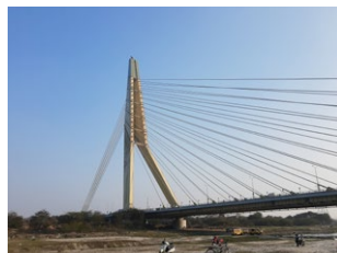
Wazirabad Bridge, India
