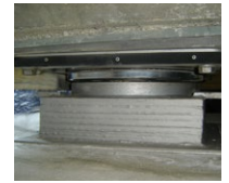
Spherical bearing
