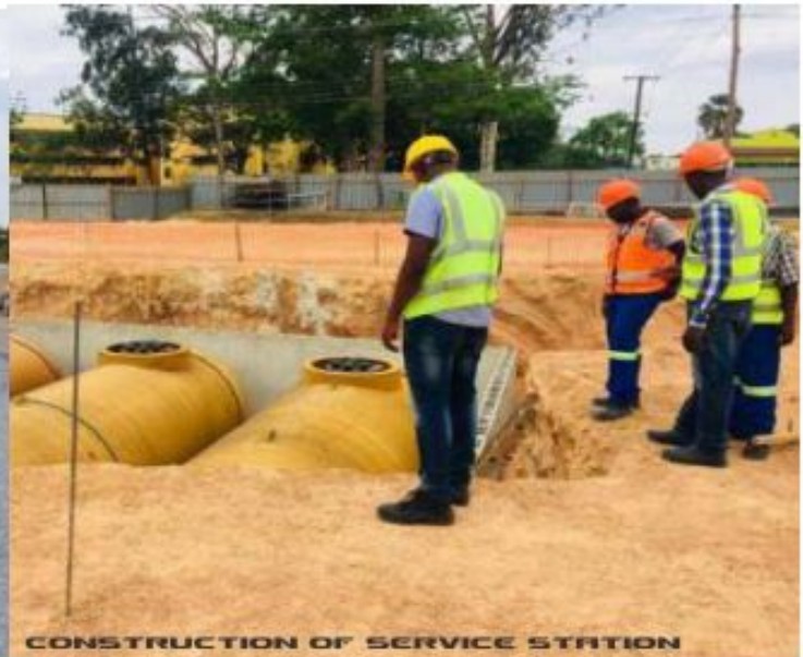
CONSTRUCTION OF SERVICE STATION
